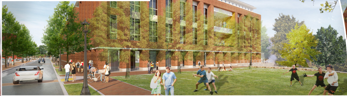
Exterior view from the southwest
